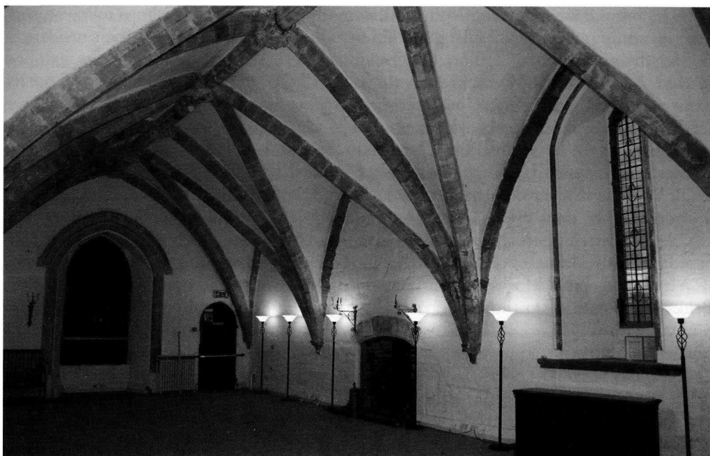
Fig. 6 (left page, top ) Undercroft RA13, looking west through the 'tunnel' through original Norman west wall to undercroft RA12. The rib-vaults here are 13th century. Photograph, A. Harris
